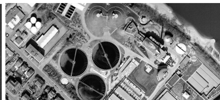
Waste Water Treatment Plant Aerial
