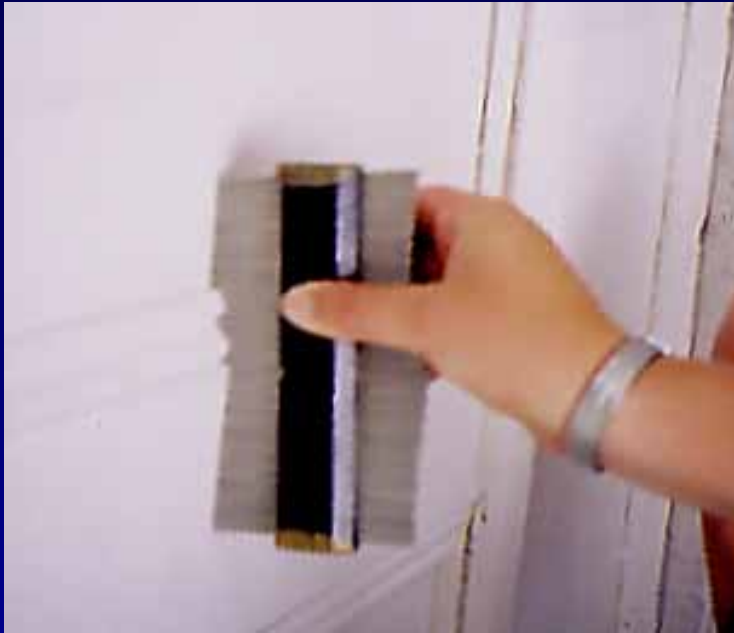
Obtaining a profile of the molding on the front door of the Mrs. Sam Houston House.
