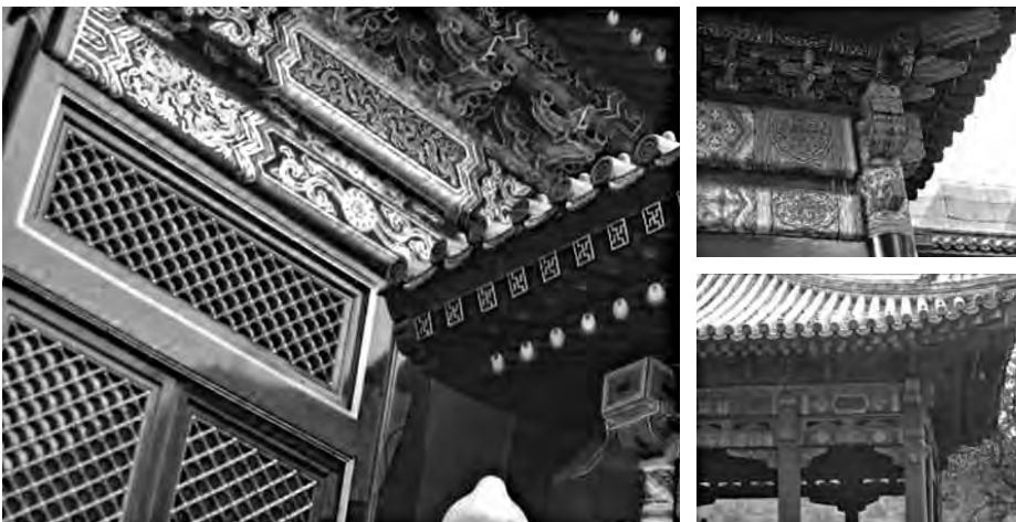
Three photos showing 'color decay' on historical buildings in the Forbidden City, Beijing: at left, a recent repainting during a major renovation of the Forbidden City before the 2008 Beijing Olympics.; top right, colors starting to decay; and below right, significant color degrading.
